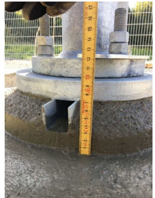
Examble of under casting
